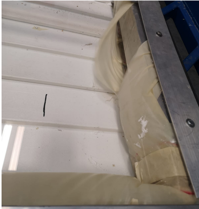
Figure 39. Failure of latex in Chamber 4; failure possibly due to latex not being engaged by weatherstripping from below the aluminum plate (weatherstripping only on right side of the angle).
