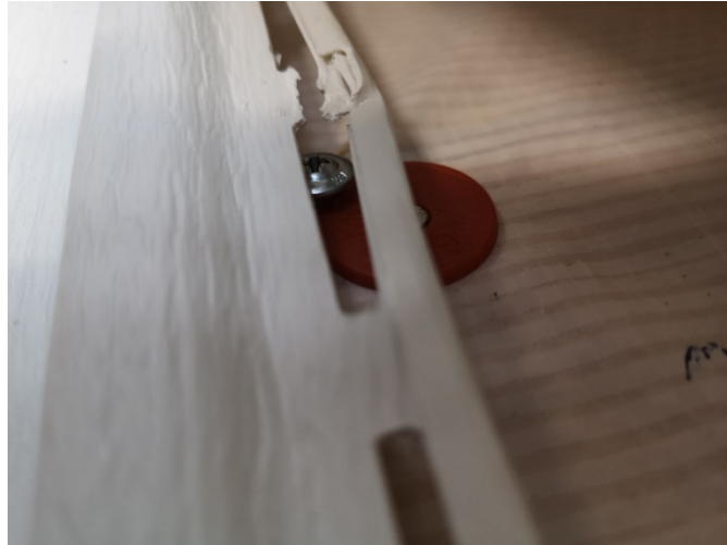
Figure 37. Detachment of vinyl siding through nail hem slots created by using punching nail. Failure occurred in chamber 3 in multiple panels.
